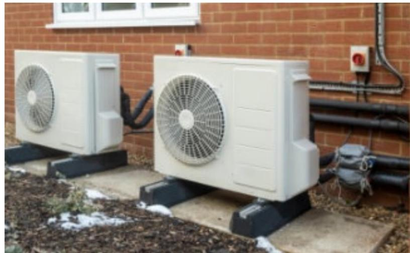
**Figure 7: An Air Source Heat Pump**
