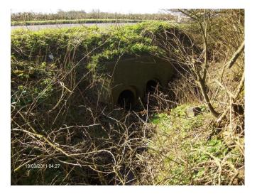
Partly silted culverts under A45
