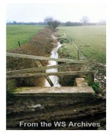
The canal bank above the brook in 1998 (Note the waterlogging to the right of the parapet)
